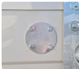
Hose lead-through (plugged) for continual feed, whilst lid remains locked.
